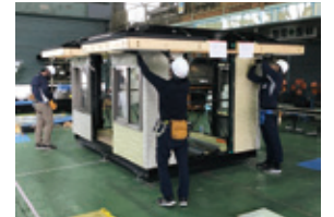
Framing/exterior course: completion test
